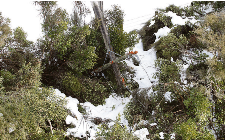
Left: pole down at Mangaweka. The recovery of downed poles may have to wait until ground conditions improve and the lambing season is complete.
